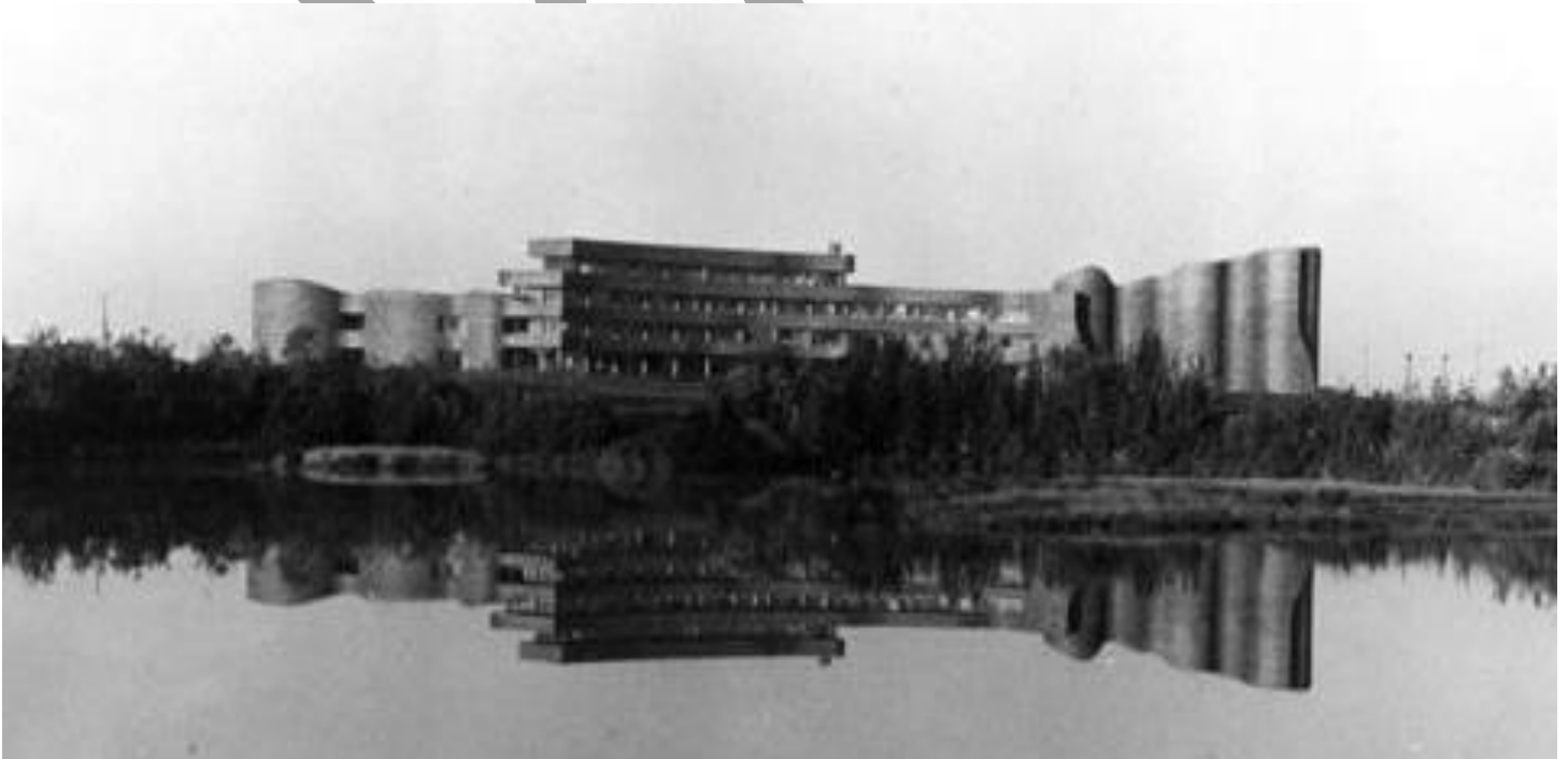
Figure 7 Grande Prairie Regional College Under Construction (1973) [South Peace Regional Archives]
